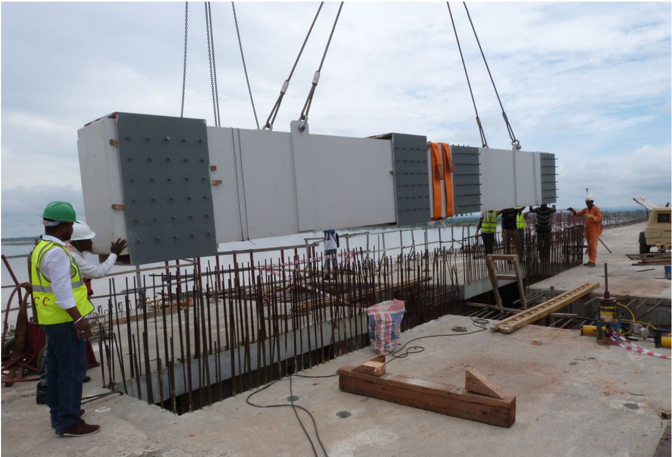
Figure 13: Insertion of steel girder into the bridge deck
