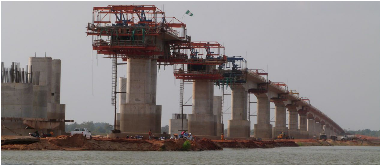
Figure 14: Work during river low level. The column shows the upper water level mark
