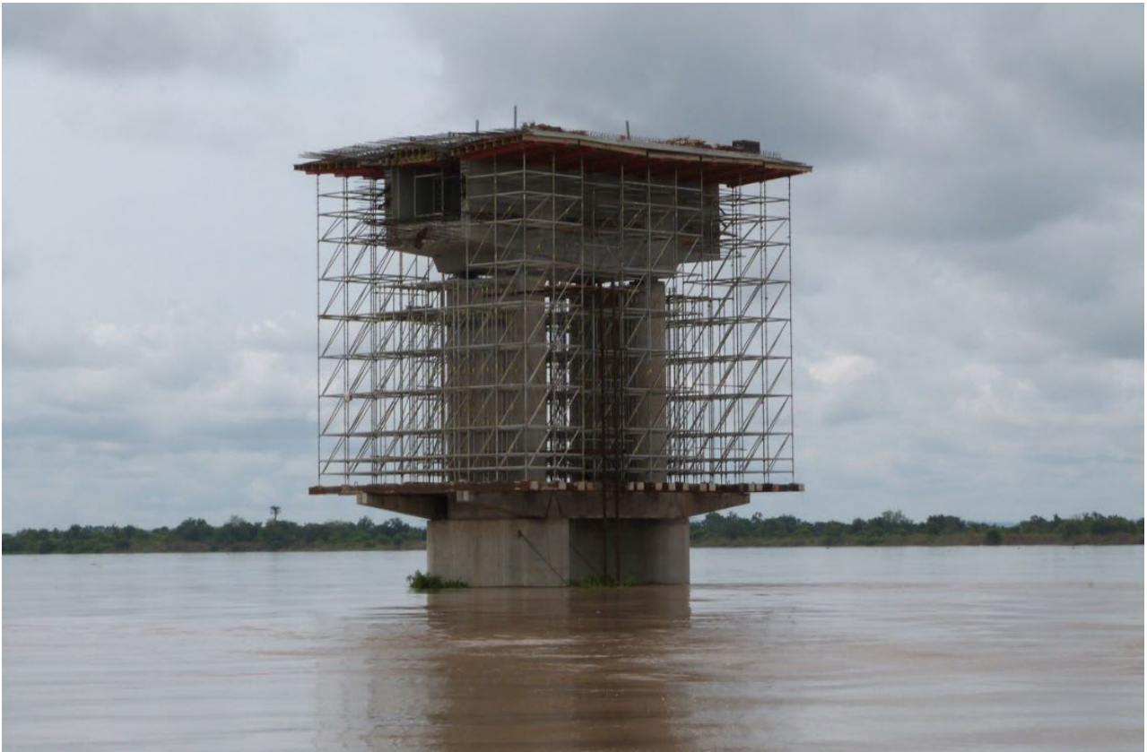
Figure 11: Temporary support girders for casting above water level
