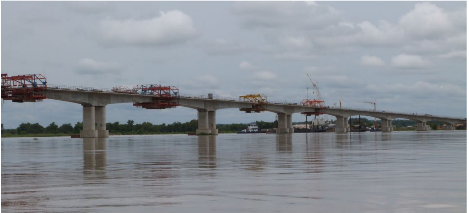
Figure 1: Construction of the Loko Oweto Bridges above the Benue River
