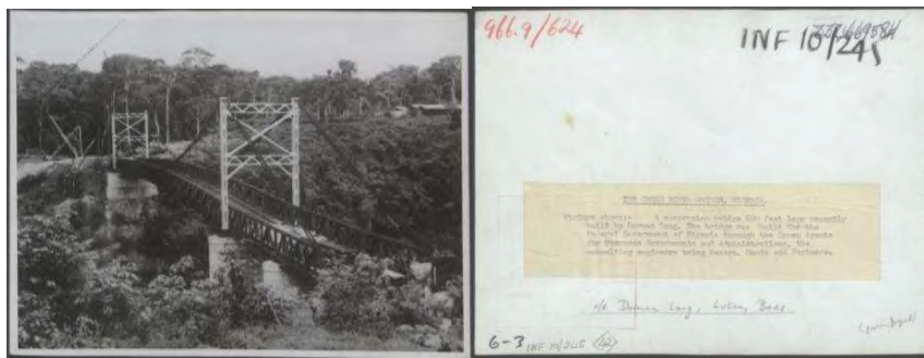
Fig. 2. Cross River Bridge during construction (Back and front of picture)
