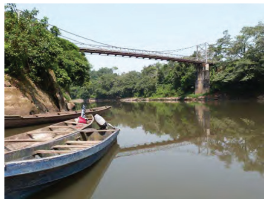
Fig. 1. Existing Cross River Bridge
